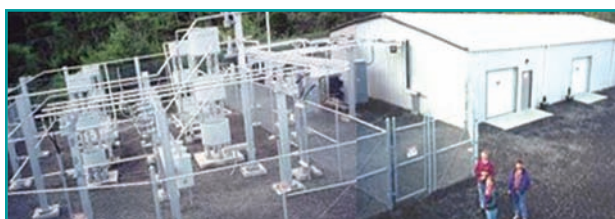
figure 5. GE/GNB and Metlatkla Power and Light battery energy storage system in Alaska. (Reprinted with permission from George Hunt, GNB/Exide.)
