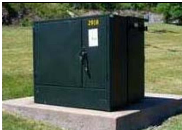
Figure 24: Pad-Mounted Distribution Transformer
