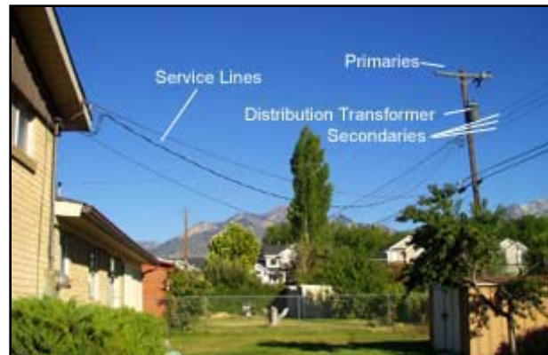
Figure 23: Household Service Line Drop from Distribution Line
